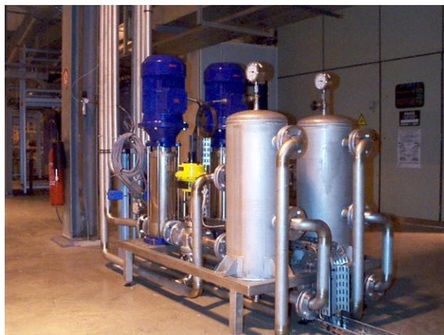
Figure 1: The new cavity temperature regulation system
