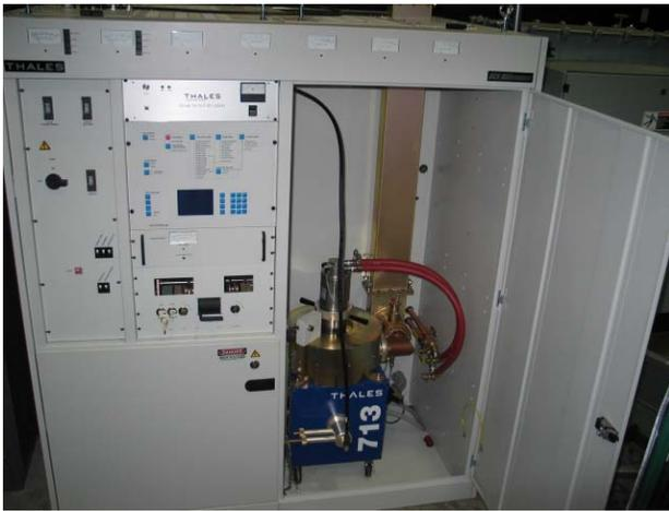
Figure 3: TH 713 IOT inside the transmitter.
