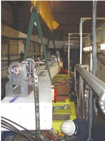
Figure 2: Installing the girder supporting the BPM3-5 triplet.
