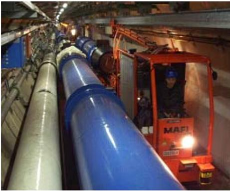
Figure 3: LHC tunnel with, from left to right: the cryogenic line, an installed and a transported magnet.
