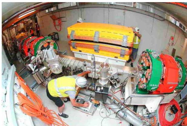
Figure 3: A fish-eye view of the installation of the final storage ring dipole magnet.
