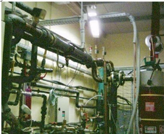
Figure 5: A view of the klystron cooling area (left side) and the 500kW, CW 5-cavity VKS-8270 Varian permanently tuned klystron (right side). The klystron has a 57-dB gain. It takes only 1 W to saturate.
