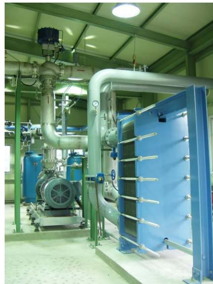
Figure 3: DTL cooling system primary loop (Pump, three-way valve, heat exchanger).
