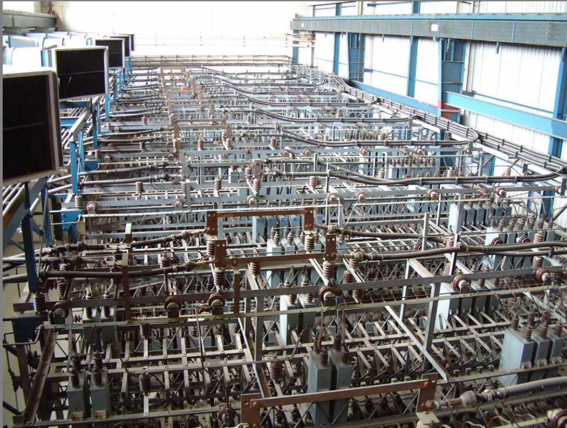
Old capacitor bank for resonating at 50 Hz with synchrotron main magnets
