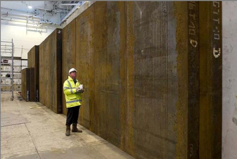
Shielding around proton beam line to TS-2
