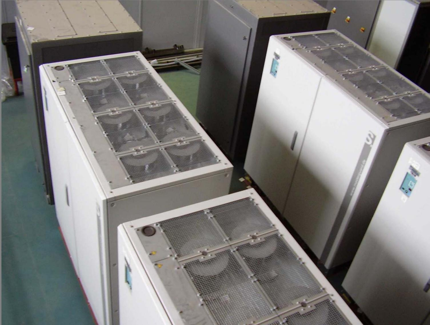
New UPSs for AC current for synchrotron main magnets
