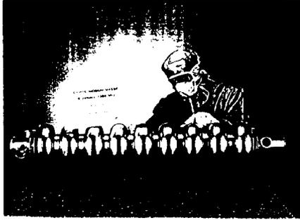
Figure 3. nine cells 1300 MHz cavity for TTF injector
