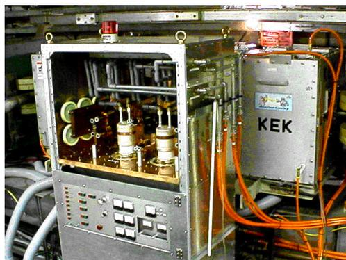
Figure 1: The MA-loaded cavity has been installed in the AGS for the barrier bucket experiment.
