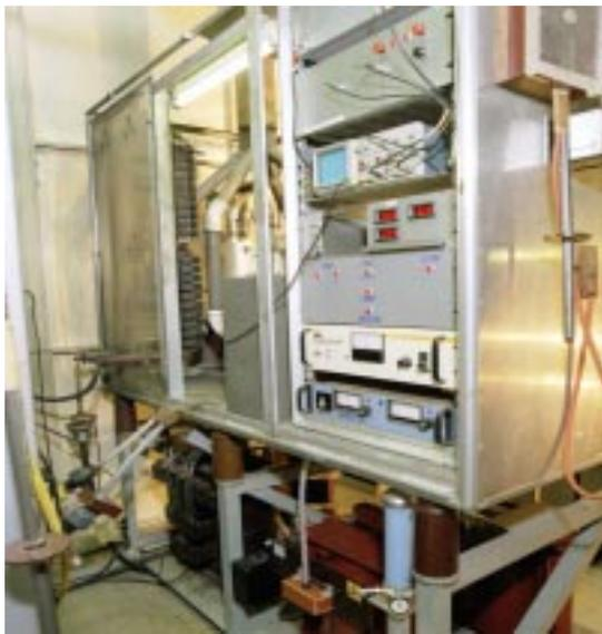
Figure 2. ISIS Linac anode modulator hardware showing the 40kV platform, CW1600 tetrodes, screen and grid power supplies and isolation transformers
