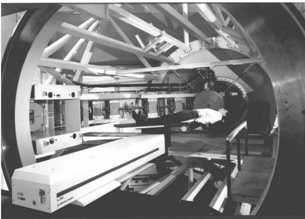
Fig. 3. Gantry and PPS under installation at the NPTC
