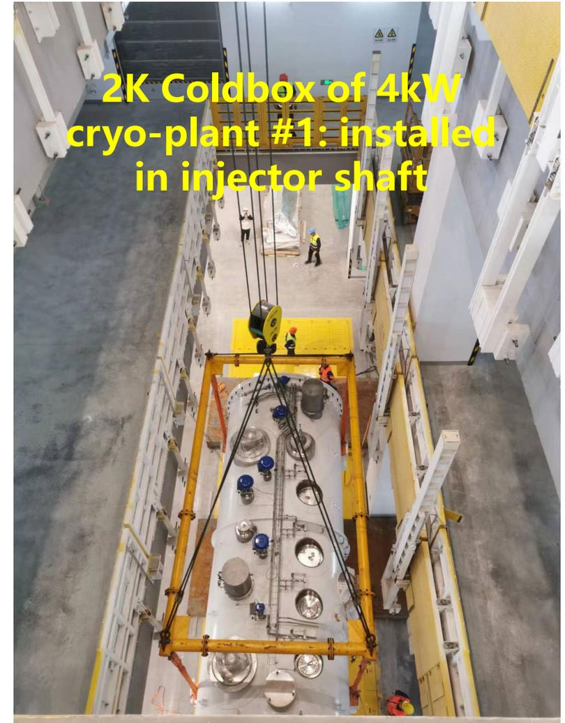
2K Coldbox of 4kW cryo-plant #1: installed in injector shaft
