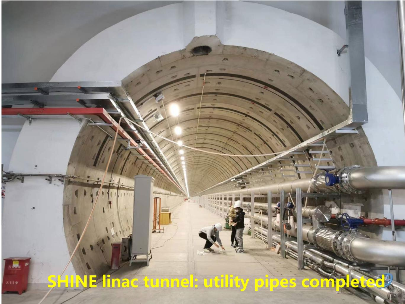
SHINE linac tunnel: utility pipes completed
