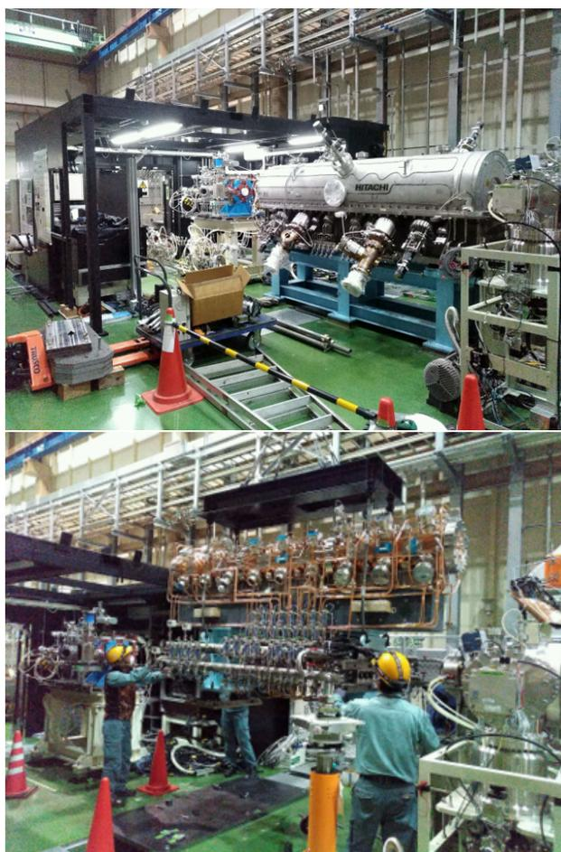
Figure 2: Decommissioning of RFQ I (upper) and installation of the new RFQ (lower).
