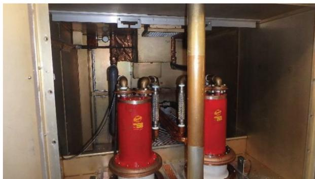
Figure 9: PA2 with stainless steel bellows.
