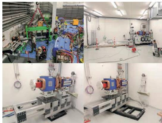
Figure 8: Status of installation of XPR optics line. Up left: XPR line in the synchrotron hall; up right: XPR room at actual state; down: scanning magnets positioned on the beam line (left) and moved out of the beam line (right).
