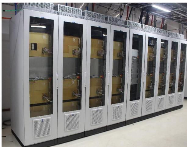
Figure 1: One of booster dipole PS.
