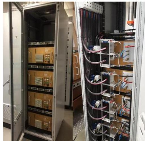
Figure 5: Front and back view of BTS quadrupole PS.
