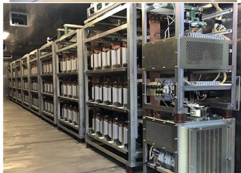
Figure 2: Pictures of power converters (upper) and a capacitor bank installed in a container (bottom) for the bending magnet family in J-PARC MR.
