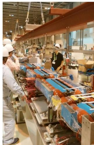
Figure 3: The 12-m LIC hung on a strong beam going to be installed inside the lower halves of multipole magnets aligned on three common girders.
