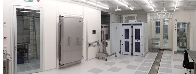
Figure 2: Photo of CR 2: the HPR with its lever for the movable wand (on top) is shown. The door of the vacuum oven and a lift trolley is shown as well.
