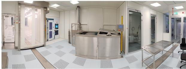
Figure 1: Fisheye perspective of CR 1. In the middle part the US and C-rinse baths are shown, on the left: Personnel air lock, roll-up door and part of the HPR.
