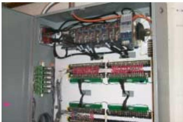
Figure 3: PLC in interlock chassis.
