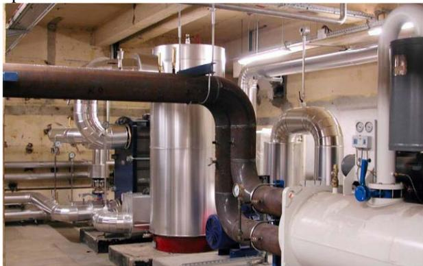
Figure 7: View of the chilled water plant connected to the RFQ temperature control system.
