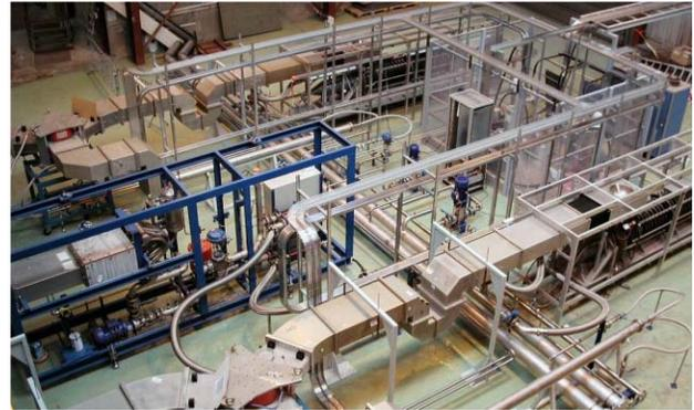
Figure 4: View of the RF power system showing the two klystron lines, the circulators and the 1.4 MW, salt water load.
