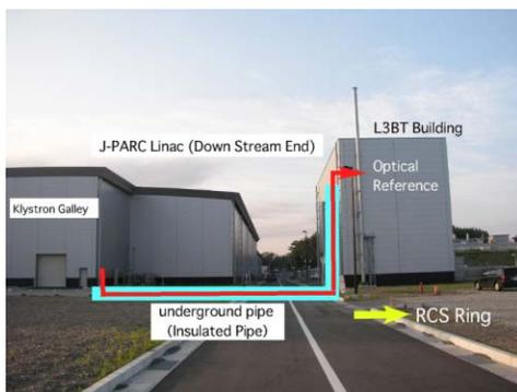
Figure 4: Passing an optical cable to the L3BT building through an insulated underground pipe
