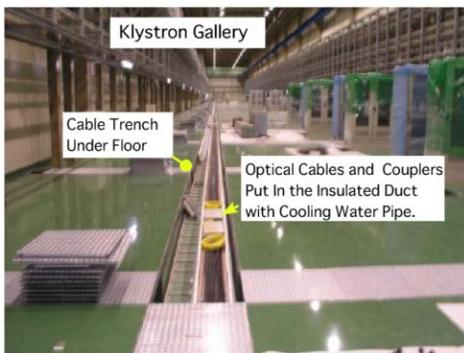
Figure 3: Installation of the optical cables and optical couplers in the insulated duct.
