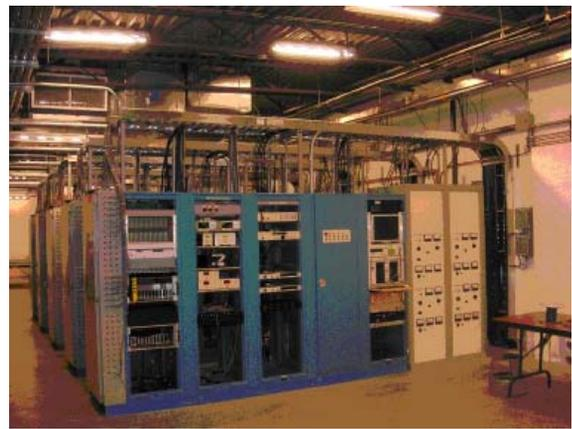
Figure 3: Installation of the service racks in the power supply room.
