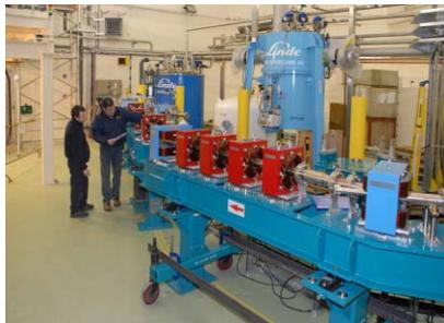
Figure 10: Installation of the 8.35 MeV transfer line.
