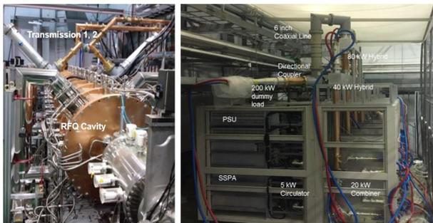
Figure 7: RFQ cavity, transmission lines and SSPAs for RF conditioning.
