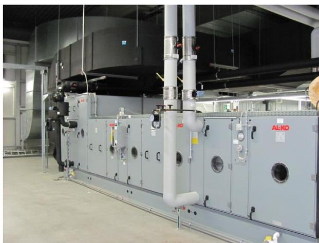
Figure 9: Tunnel Air Handling Unit.
