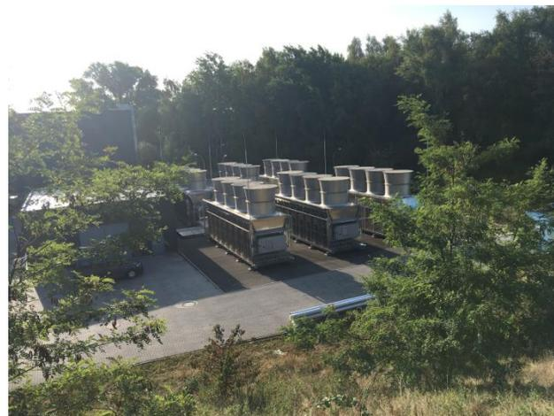
Figure 4: XHM cooling towers for dry and wet cooling.
