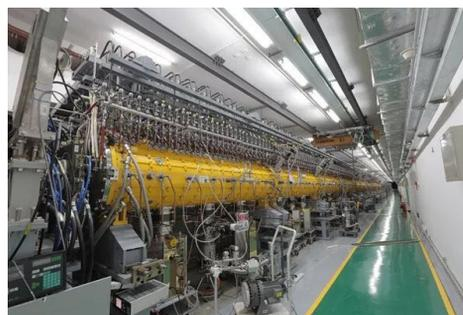
Figure 1: The CSNS DTL in tunnel.
