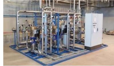
Figure 5: RFQ water-cooling skid installed at ESS.
