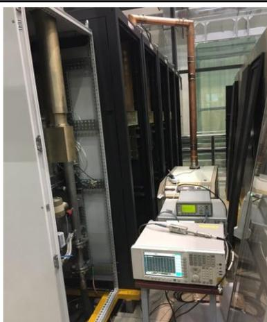
Figure 2: 325 MHz/25 kW SSA.
