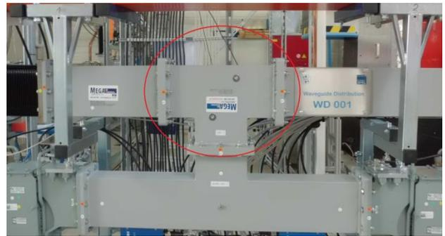
Figure 5: Asymmetric shunt tee of a waveguide distribution.
