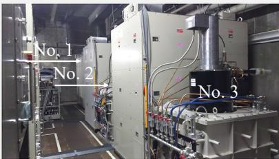
Klystron and power supply unit (x3)
