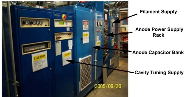
Figure 3: Layout of the support power supplies for Station RF-11
