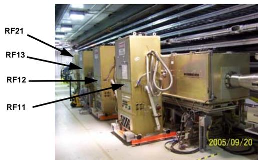
Figure 2: Cavities and Amplifiers installed in the SNS Accumulator Ring tunnel.
