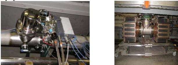
Figure 3: 201-MHz section soft vacuum 8" cryopump (left) and 1200 L/s ion pumps (right).
