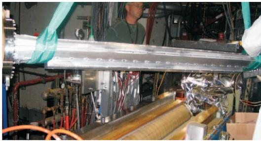
Figure 9: New HER Q5 chamber during installation.
