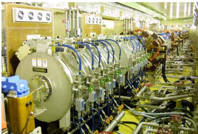
**Figure 4:** Ten RF systems installed in the RCS tunnel.
