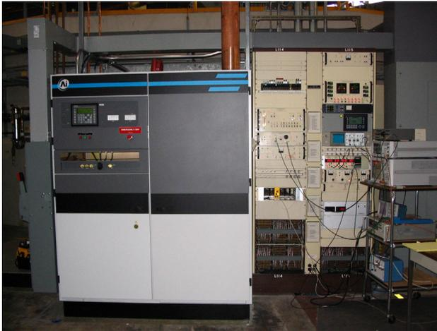
Figure 2: HPA installed at ALS.
