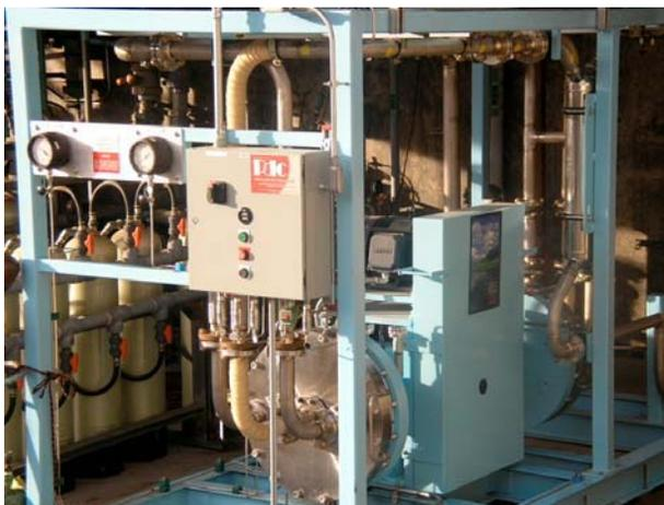
Figure 3: Skid-mounted compressor for SF<sub>6</sub> recycling
