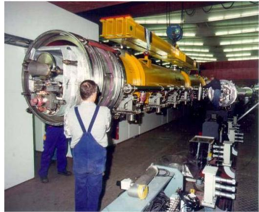
Figure 3: Installation of a FLASH accelerator module.
