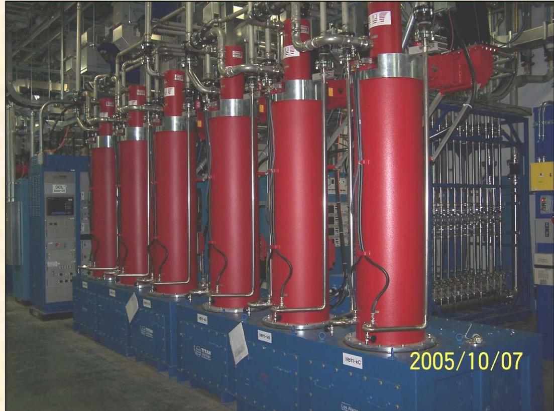
Each high-voltage power supply supports 11-12 klystrons.
