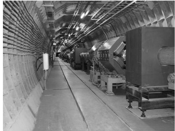
Figure 1: Section of PRGC-100 with quadrupole lenses and radiation protection blocks.
